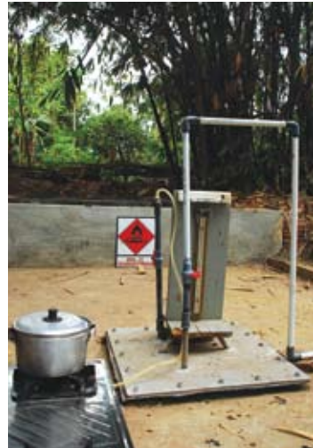
Fixed Dome Anaerobic Bio-digester at PT YTL Jawa Timur's TK- 4 Station
