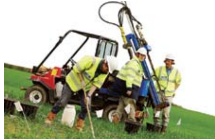
Staff conducting soil tests as part of Wessex Water's catchment management work
