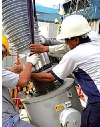
High Voltage Transformer Bushings replacements being carried out
