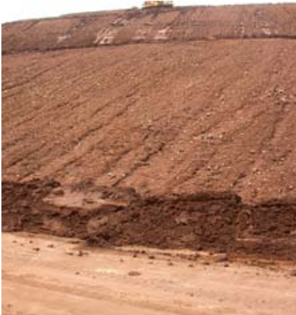
Before: Ash Disposal Area (original condition)
